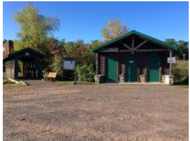
The wetland park committee prepared a grant application and presented it to Louisiana Pacific Corporation in 2008. This grant provided the funds used to construct the handsome public restrooms pictured above.
