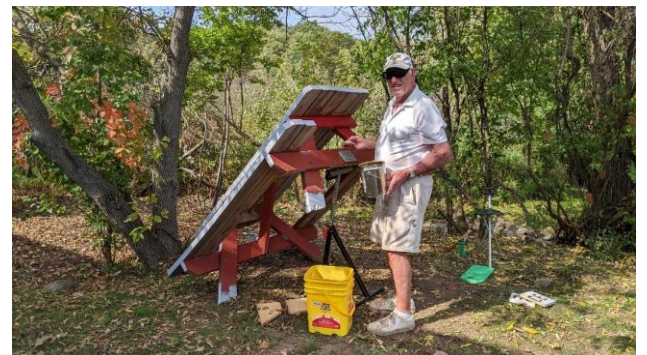
Tom McDonnell working on the Wetland Park picnic tables to get them ready for spring. Some of them needed new boards; and some of them needed partial re-staining.
